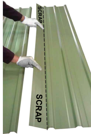
Fold middle section of sheet until free
