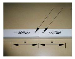
Finished Channel. The joined channels should now look like the picture with the CSJ positioned equally inside of the joined channels. Drill out holes with 3mm drill bit in CSJ to match the holes in channel. Drilling of screws on the joined channels is being done after sheets are locked on the spliced channels.
