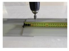
Step 3. Turn over the ridge beam. Measure 250mm from the middle along the centre of one ridge beam, mark spacings of 50mm. Fasten with a Tek screw at each marking.
