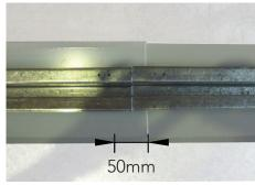
NOTE. There is a 50mm overlap of the ridge caps when the beams are in position.
