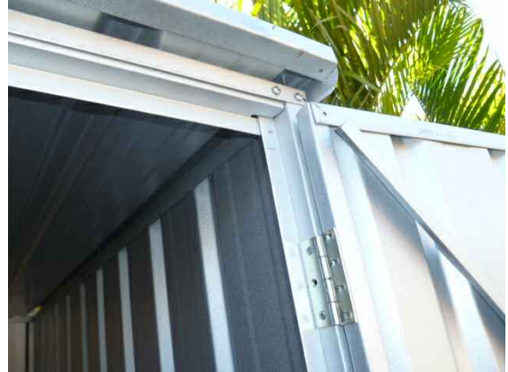
DOOR CONNECTION & JAMB ASSEMBLY
